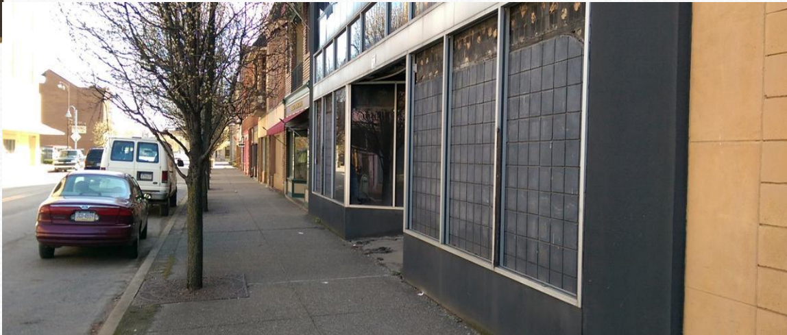
Blocked Building Facades
