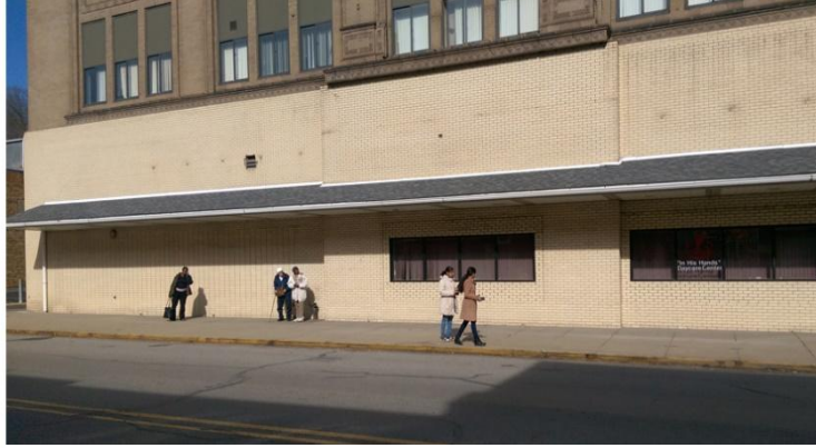
Absence of a 'Bus Stop'
